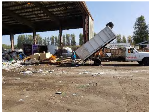
Figure 18: South Side View of Transfer Station
