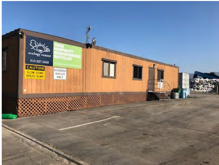
Figure 41: Facility ID Sign for Ecology Center
