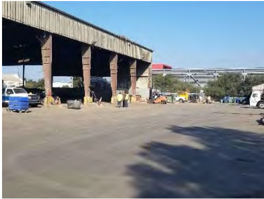
Figure 6: Transfer Station Building
